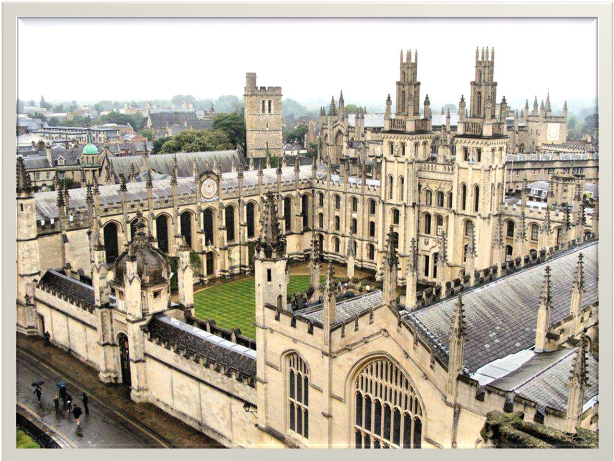
Oxford University, England Walls waterproofed on the interior, using Tecmadry-F
